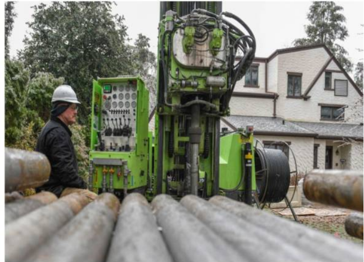
Geothermal heating system installation in Scarsdale, NY
