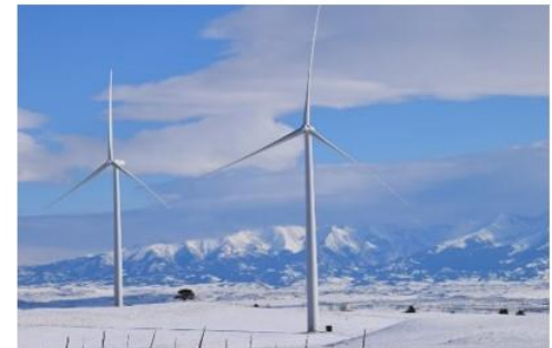
Big Timber Wind Project - Located in Montana
