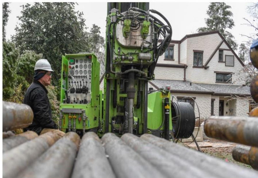
Geothermal heating system installation in Scarsdale, NY
