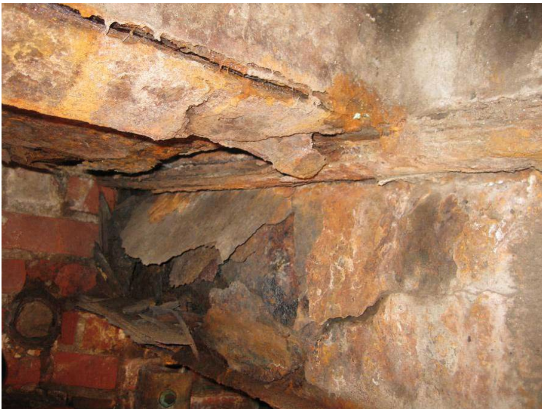
Figure 2: Corroded beam
