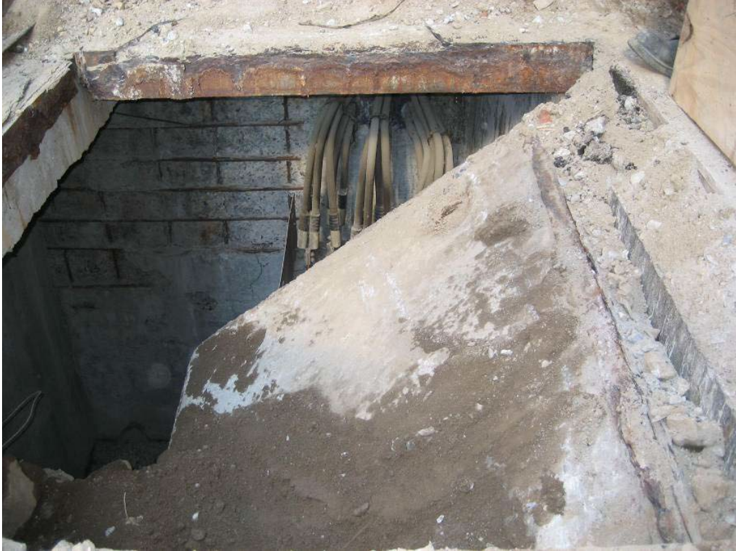
Figure 1: Collapsed roof
