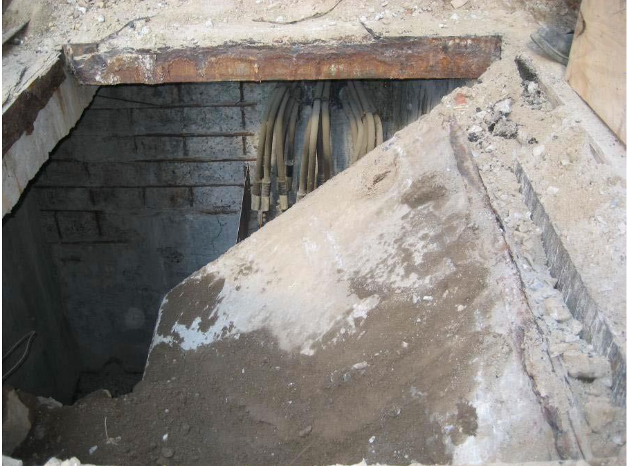
Collapsed Roof
