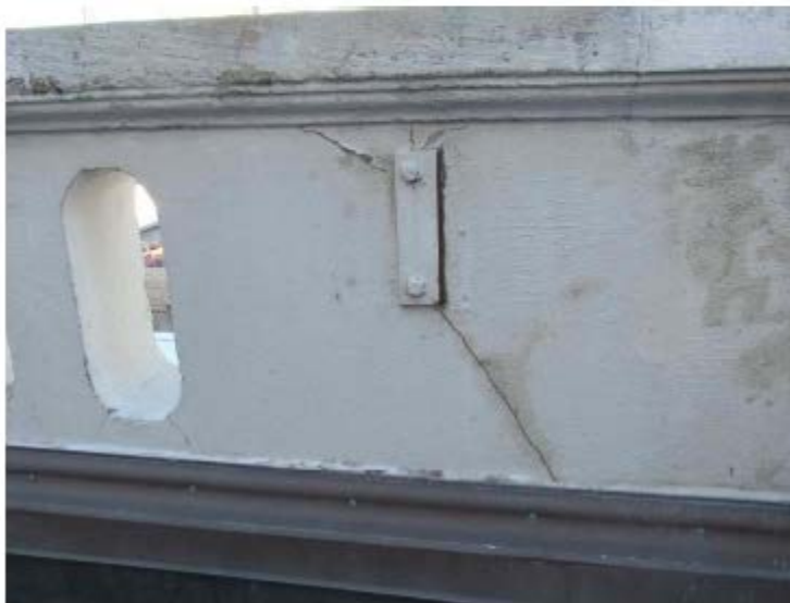
Photo: P098 Date 9/25/2017
