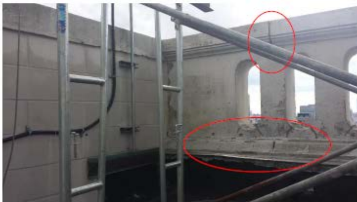
Photo: P100 Date 9/25/2017
