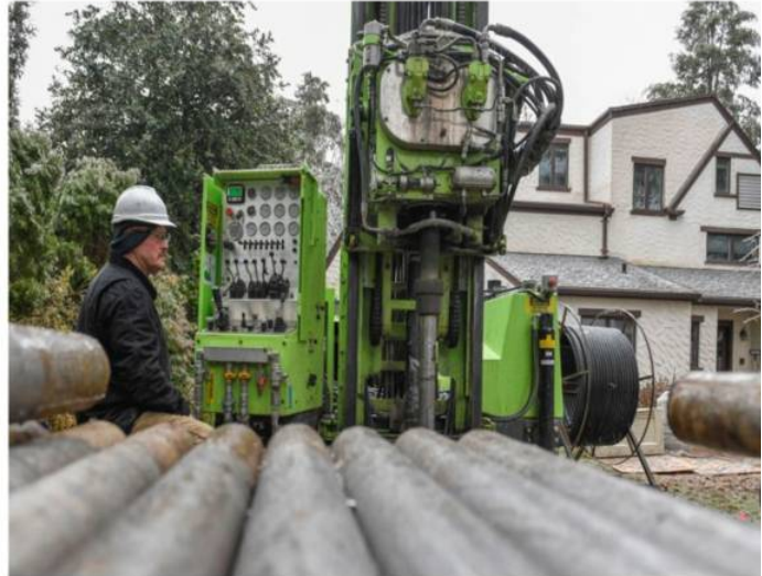
Geothermal heating system installation in Scarsdale, NY
