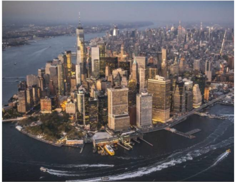
CECONY's steam system provides environmentally-friendly energy from the southern tip of Manhattan to 96 th Street
