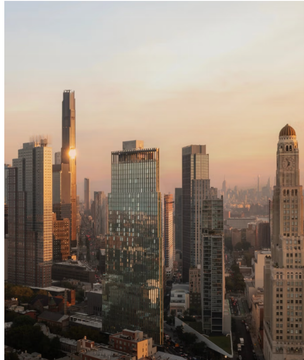
All-Electric Skyscraper at 505 State Street in Downtown Brooklyn is 100% electric and carbon neutral
